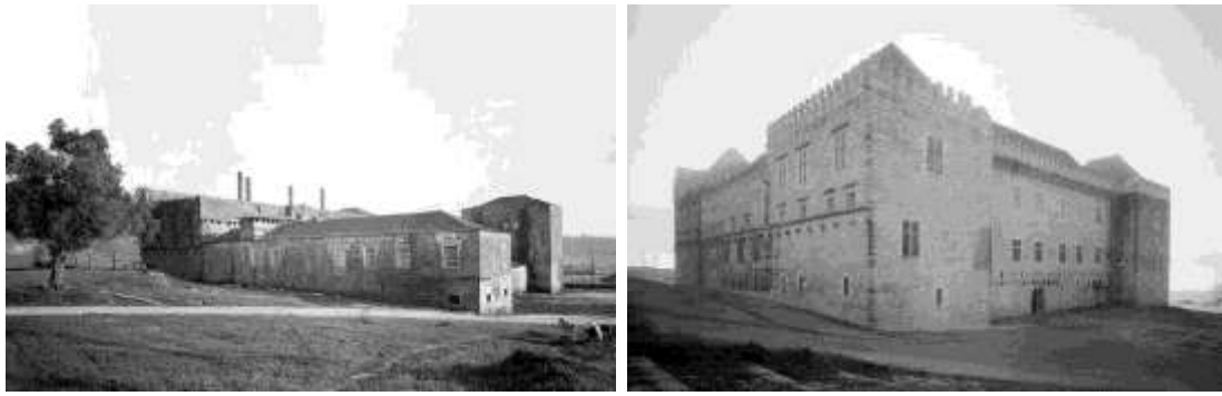
figures 23 and 24: Palace of the Dukes of Bragança in Guimarães, before and after the intervention in 1940
