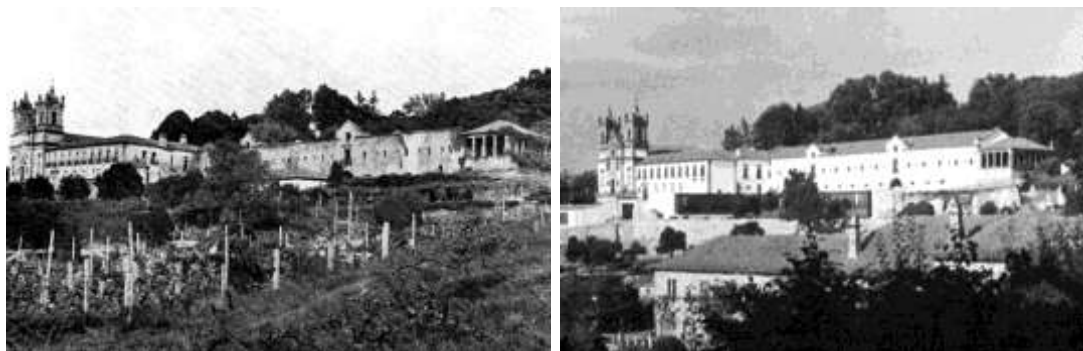
figures 12 and 13: the former monastery of Santa Marinha da Costa in Guimarães, before and after the reconstruction of the new wing rooms, 1985
